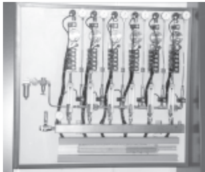
Distribution panel 6 lines
