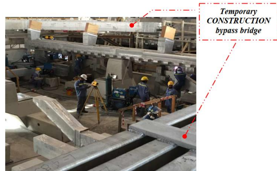
Figure 8. Installation of new busbars and supports.
