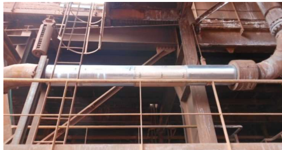
Mineral wool used inside the plant
